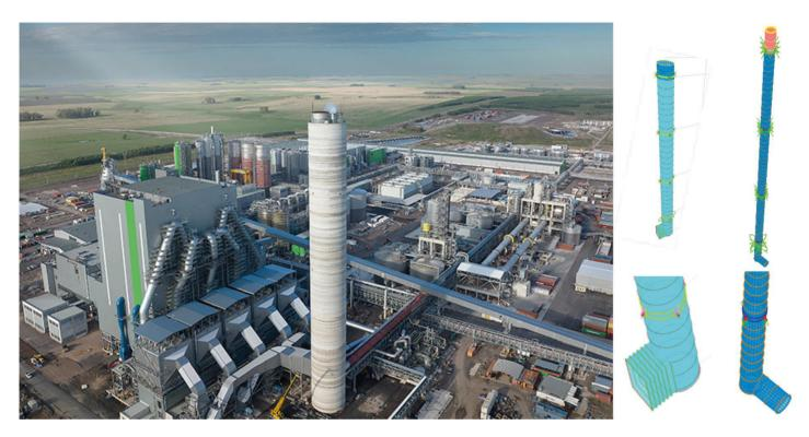
Design of 6 steel stacks for the new cellulose plant of UPM at Paso de los Toros, Uruguay in 2023. With a capacity to produce 2.1 million tons of eucalyptus pulp per year, the mill is the biggest in Uruguay and the world's biggest single line mill in operation. It will also contribute around 1 TWh of surplus green electricity per year to the Uruguayan power supply
